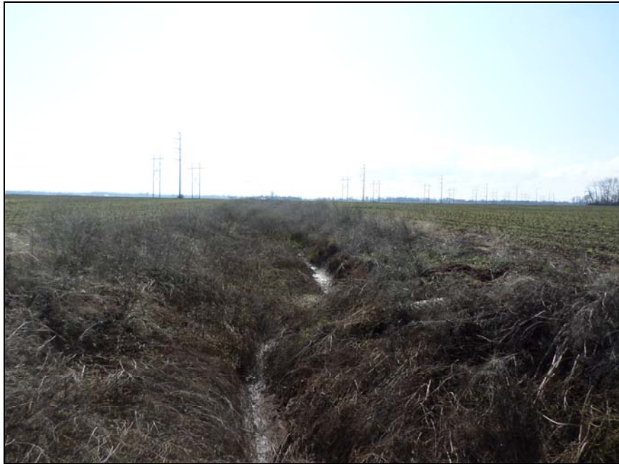
Western-most farm ditch facing south from outfall
