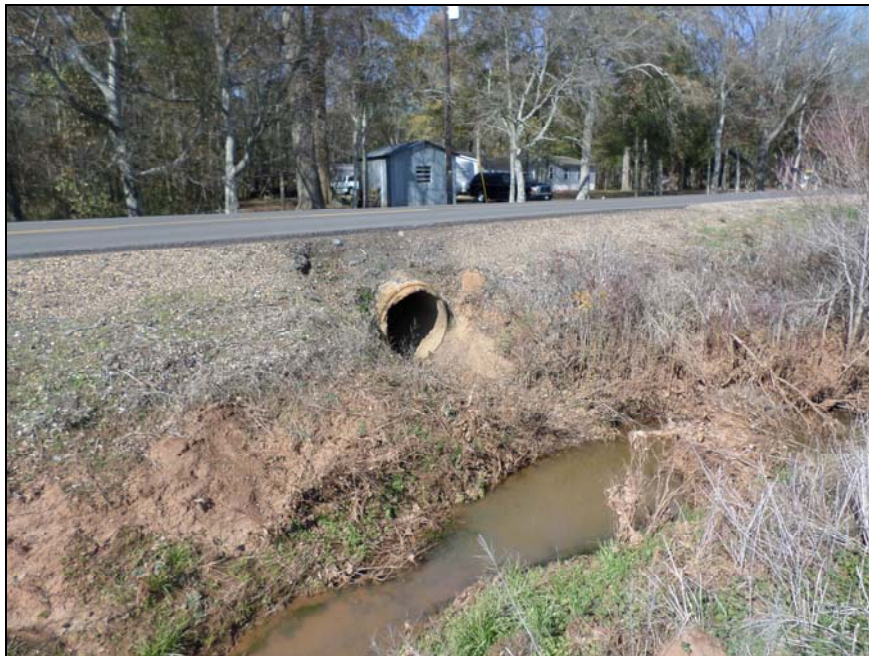
Intermittent stream/culvert at Rapides Station Road
