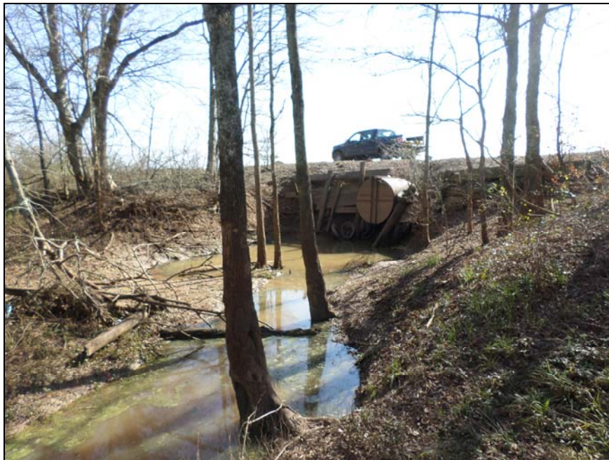
Data Point #1 facing outfall/culvert from ditch
