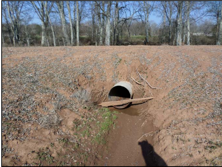
Culvert at Farm Ditch/Big Bayou
